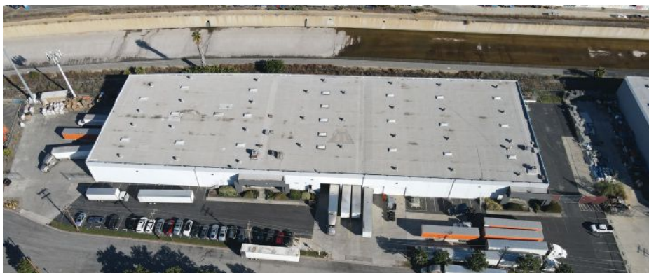
Located at 14313-14351 E. Bonelli Street in the City of Industry, the property features 69,498 square feet of multi-tenant distribution space.
