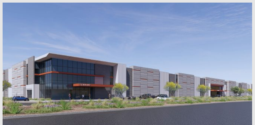
The Block on Elliot will be a 270-acre industrial mixed-use development project on the site of a former dairy farm in Mesa, Ariz.
