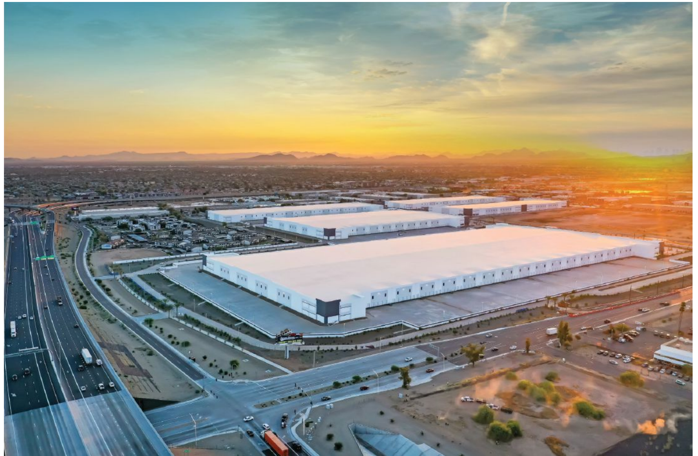
Colson Group USA leased 118,833 square feet at West 202 Logistics. The manufacturer and distributor of caster, wheel and related hardware products will occupy the space late last year.
