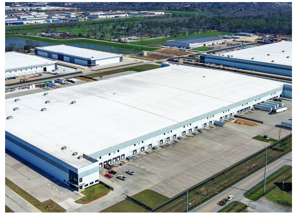
Kennedy Greens Distribution Center Houston. Photo courtesy of CapRock.
