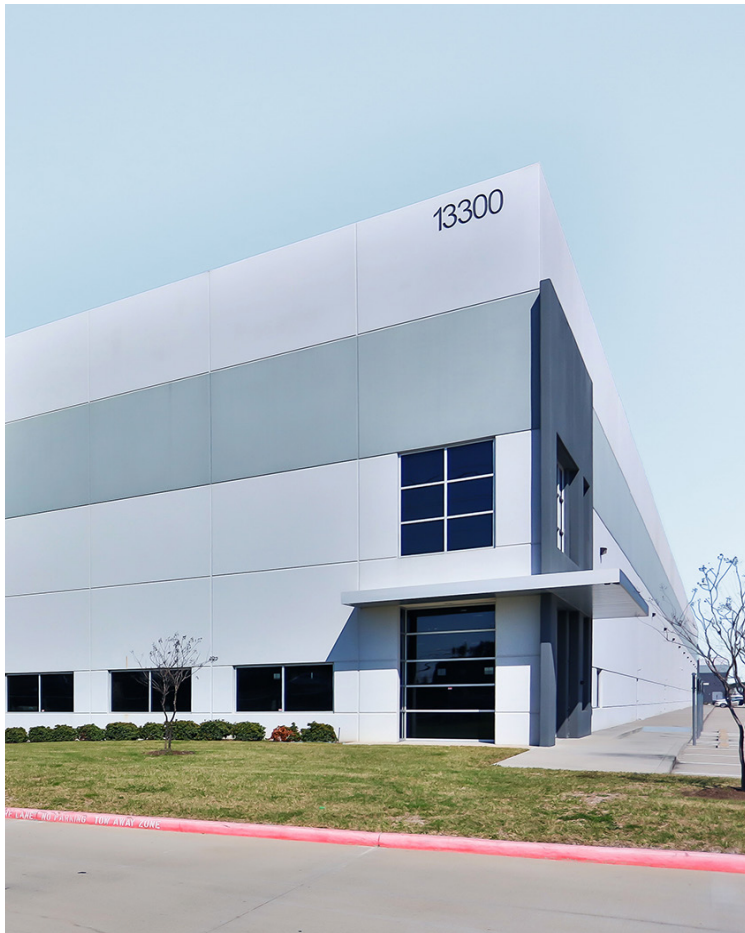
Kennedy Greens Distribution Center Houston. Photo courtesy of CapRock.
